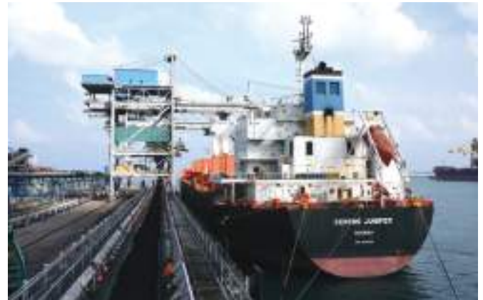
Common user Coal Terminal – 1
