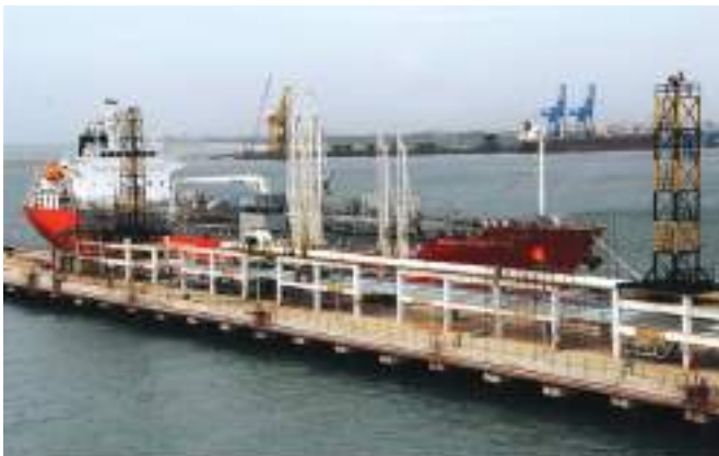
Marine Liquid Terminal
