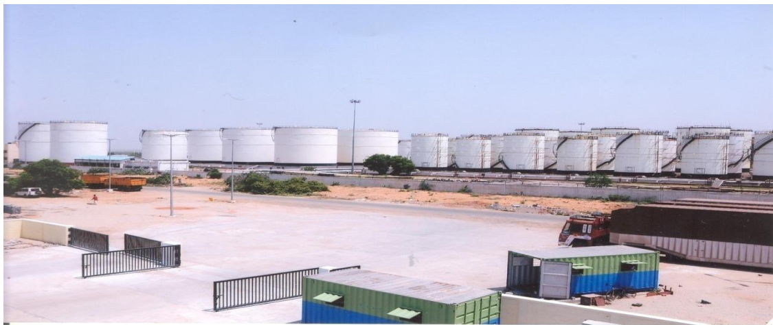
Fig. 4 - View of Tank Terminal
