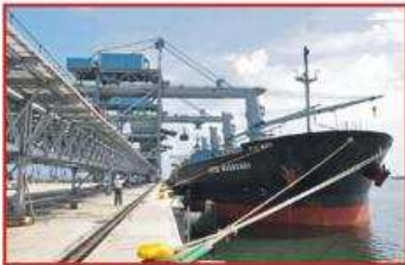
COAL UNLOADING AT CICTPL TERMINAL
